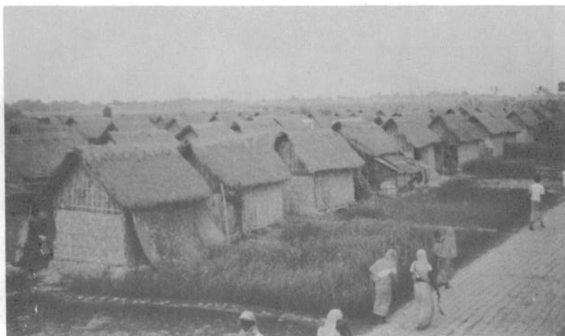
Plate 18: Sites and Services - A squatter resettlement scheme where building materials are provided by relief agencies in Dattapara, Dacca.
