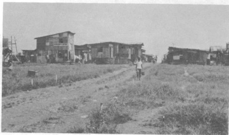
Plate 16: Transit and Relief Camps - The Makati Health Centre Relocation Area in Taguig, Manila, where water is supplied by fire trucks.
