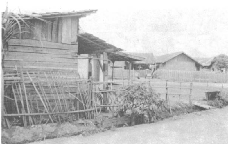
Plate 10: Purchased Houses - Houses purchased in cash by low-income families, Klender, Jakarta.
