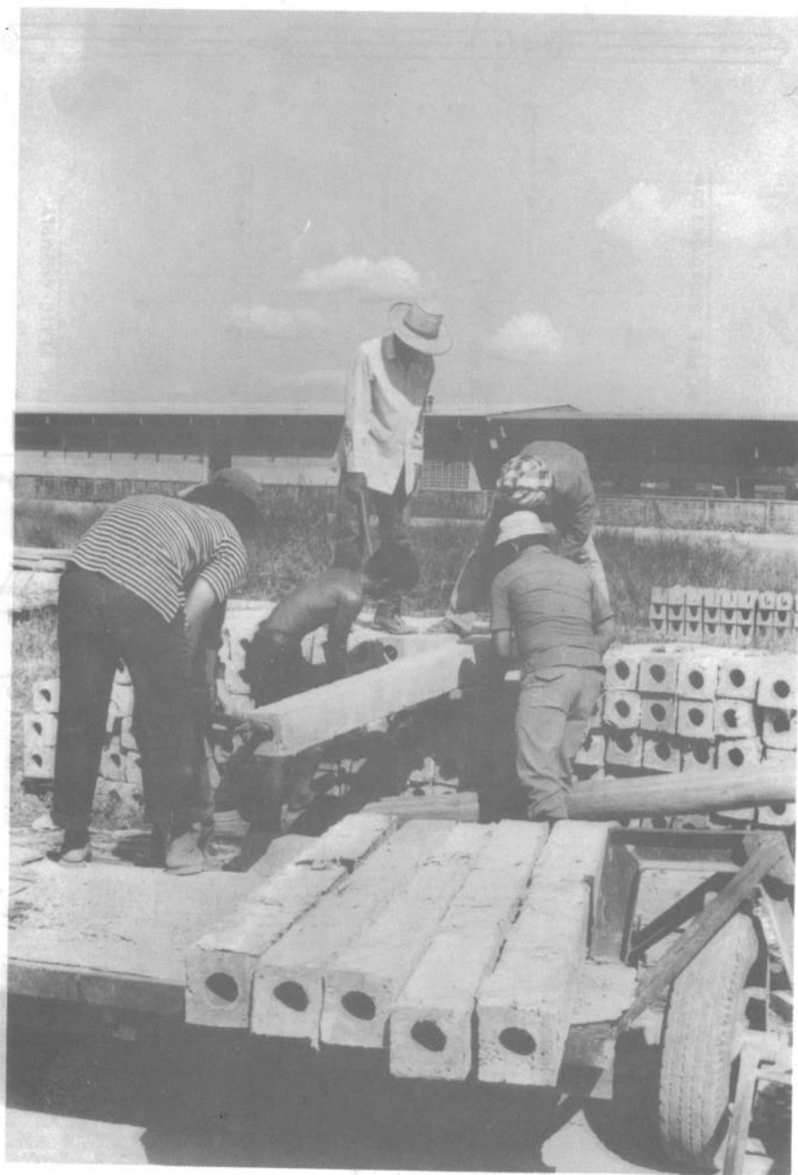
Plate 2: Short piles being unloaded on the site.
