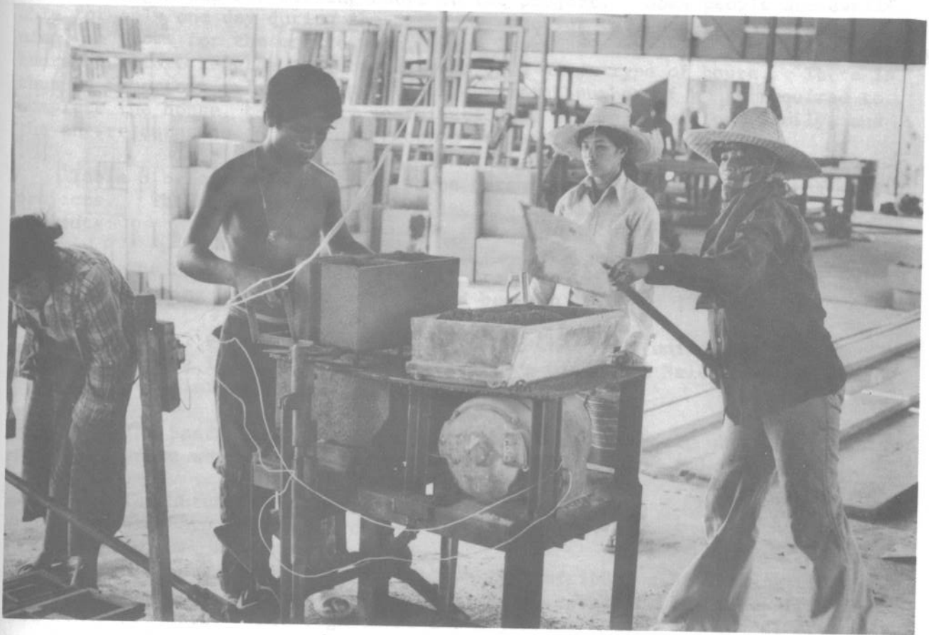
Plate 5: Block making team in action. Women pouring mixture and operating the block machine and man carrying blocks to drying area.
